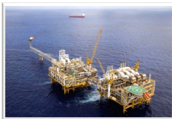
Figure 6: Bayu Undan Facility
